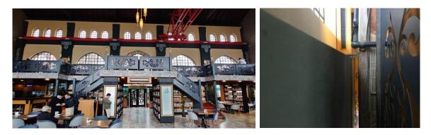
Figure 10. Mezzanine floor and masonry structural wall (Torunbalcı archive, 2019)
